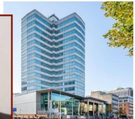
Hodge House 1960s headquarters
