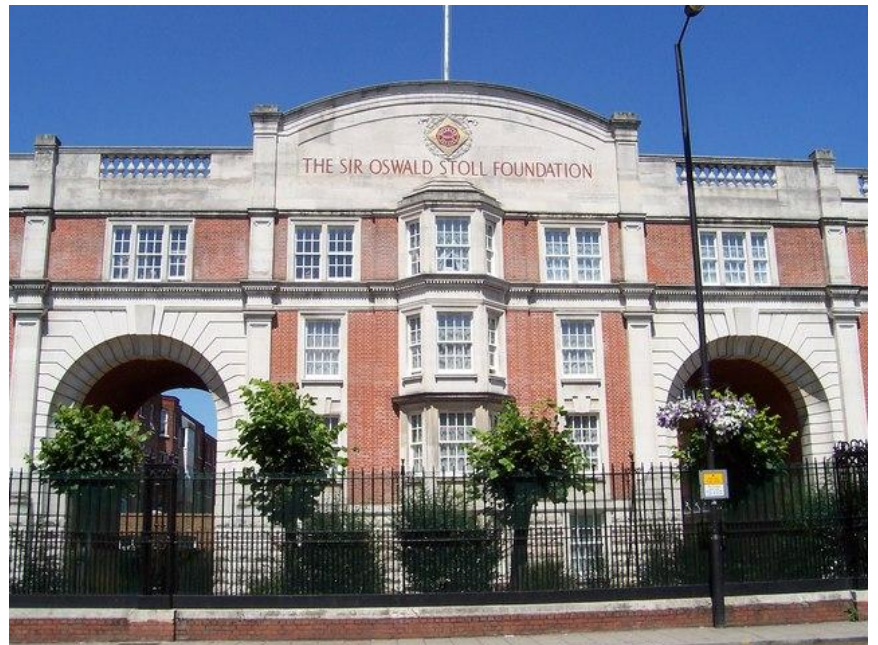
The Sir Oswald Stoll Foundation Headquarters in Fulham
