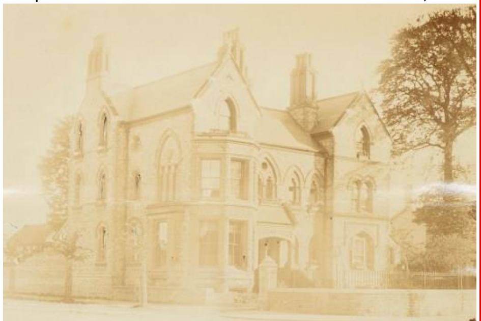
A rather faded late 19 th C view of Howard Lodge, 28 Newport Road Credit: Glamorgan Archives
